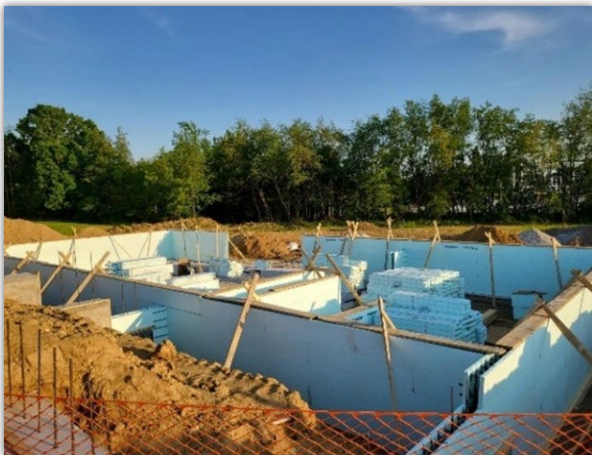
Grace Baptist's new foundation
